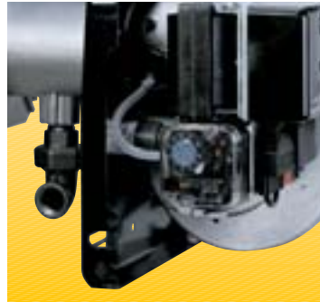
Air pressure switch
